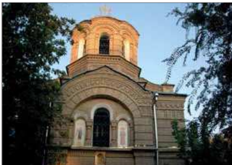
Fig. 68. The Church of Christ the Savior, built in 1878, is surrounded by trees and numerous shops of the local bazaar.
