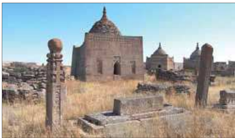
Fig. 83. The Seysen Ata cemetery complex contains funerary monuments dating from the 14th to the late 15th century.
