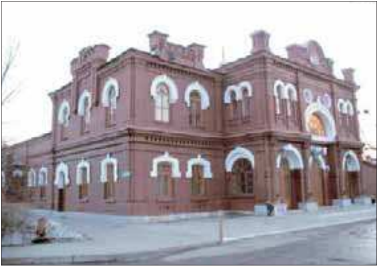
Fig. 104. The Zhambyl Theatre of Ust'-Kamenogorsk is more than a hundred years old.
