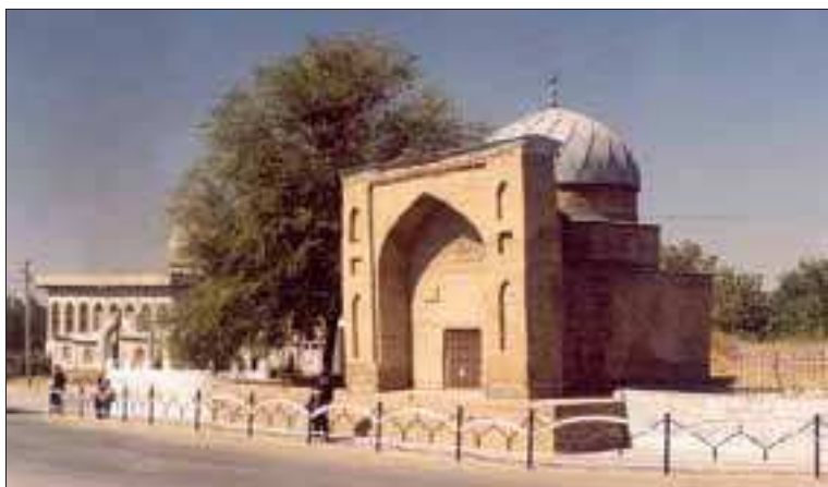
Fig. 63. The Mausoleum of Karashash Ana is an architectural monument dating from the 13th–14th century, built over the grave of the mother of Khwaja Ahmad Yasawi.
