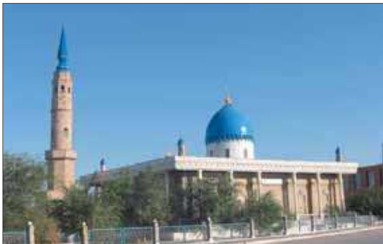
Fig. 67. The Aytbay Mosque, probably the most important monument in Kyzylorda.
