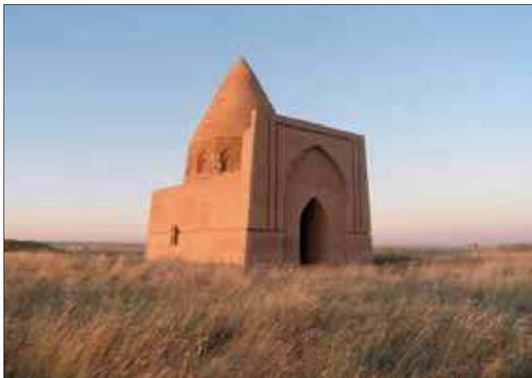
Fig. 92. The name of the cemetery, Abat Baytak, comes from a building that is a fascinating example of a baked-brick mausoleum with a conical covering, one of the rarest to have survived to the present day.
