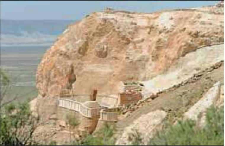
Fig. 82. Beket Ata is one of the cemetery complexes with an underground mosque that is most representative of western Ustyurt.
