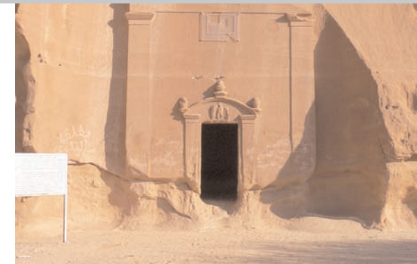
Ph.58: Eolic erosion on a al-Khuraymât façade (detail), S. Ricca, 2006.
