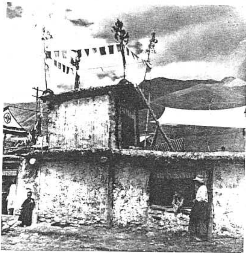
13. Tree-branches, rags and 'wind horses' on the roof of a house (note the ladder, a notched tree-trunk). Photo: V. Sís/J. Vaníř.
